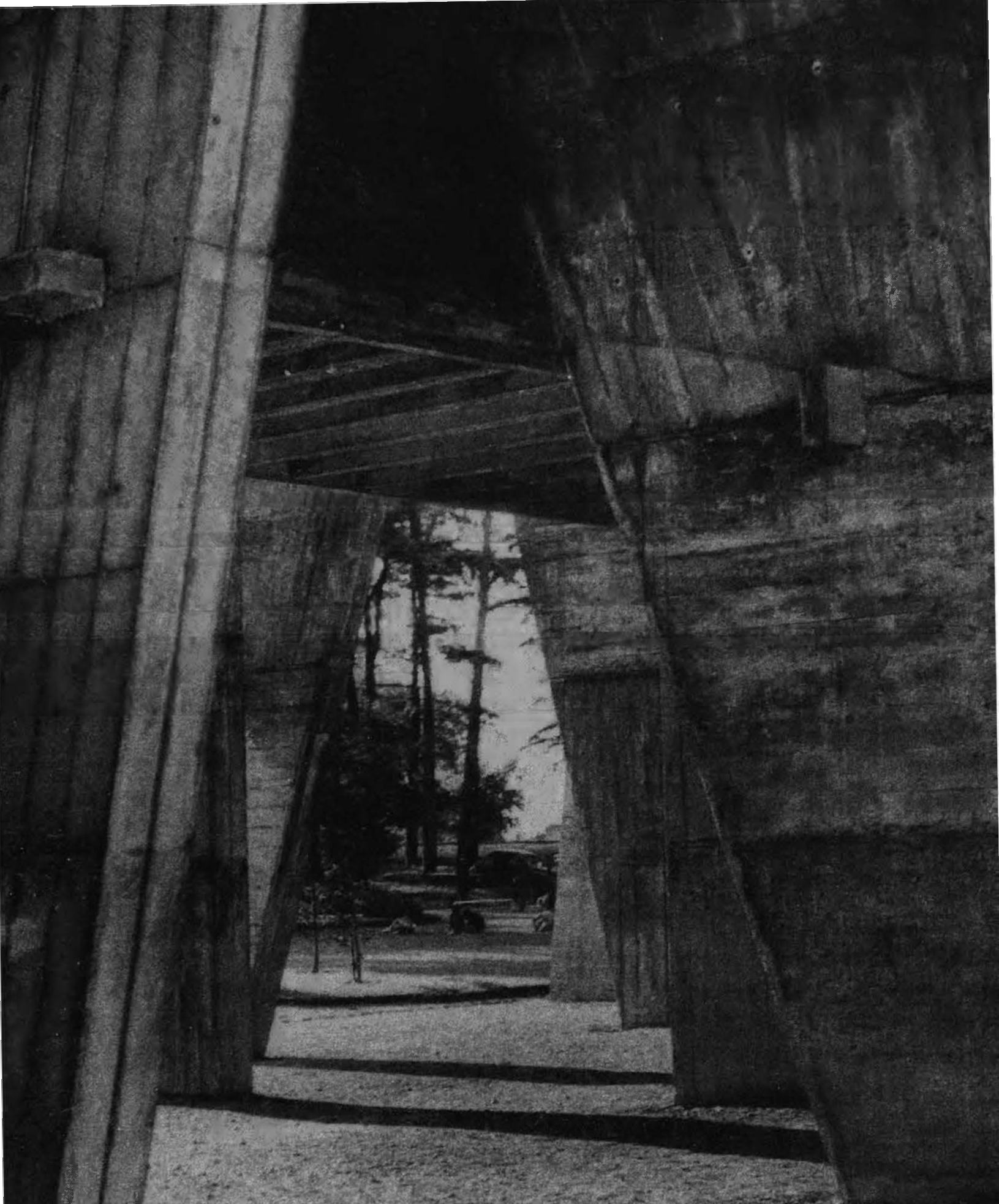
Figure 8 Le Corbusier, main street on columns, Unité d'habitation in Nantes, 1952
